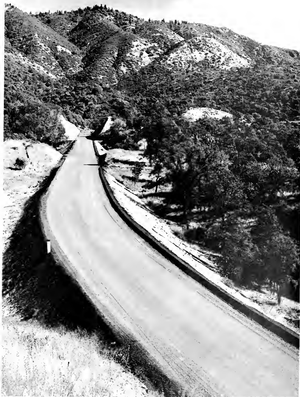
New unit on recently completed realignment of State Highway section between Squaw Valley and Dunlap on Kings River Canyon Highway
